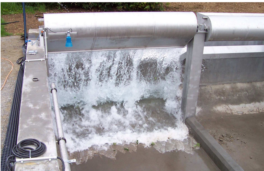
Figure 3: Flushing tipping flusher (test run)
